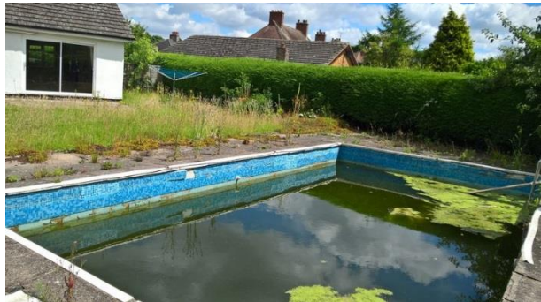
Plate 9.4: Swimming Pool to the Rear of No. 80 Tatenhill Lane.
