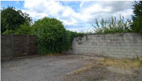
Plate 9.3: Boundary Features (Breezeblock Walling and Wooden Fencing) at No.80 Tatenhill Lane.
